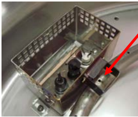
Pilot Window lined up with burner hole.
